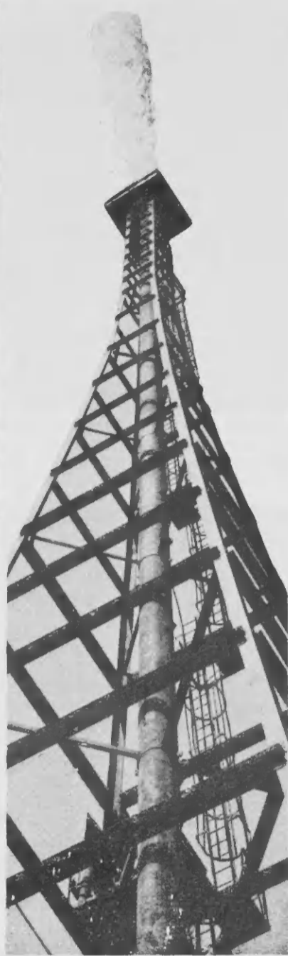
ALKY-2 FLARE is the refinery structural giant, standing well over 200-feet high.
